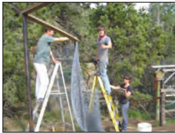
Fence building and maintenance is an on going project
